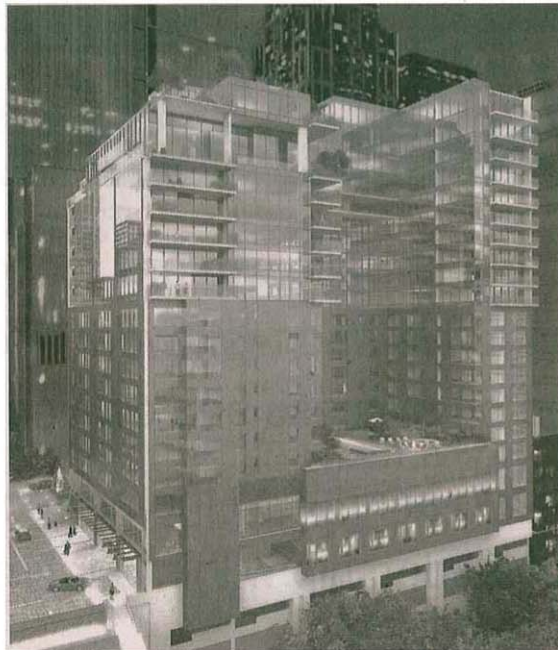
The Four Seasons Hotel and Private Residences Seattle , now under construction, will have 149 rooms and 36 condominiums. Two-thirds of the condos have sold at nearly $2,000 a square foot.
