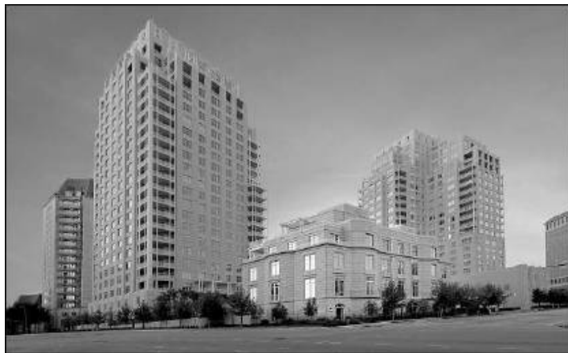
Four Regency Row townhomes are complete at the master-planned Ritz-Carlton neighborhood. They are priced from $4.5 million.
